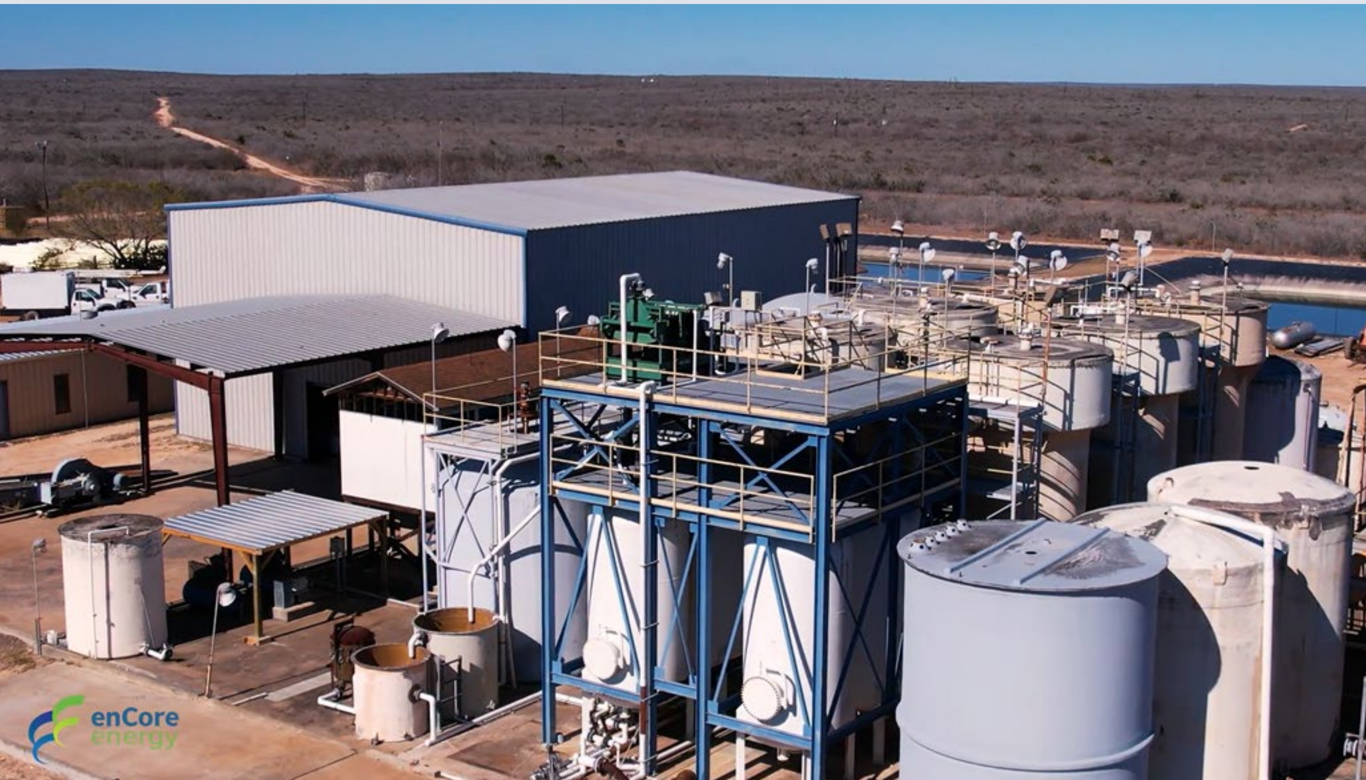
Rosita ISR Uranium Processing Plant
