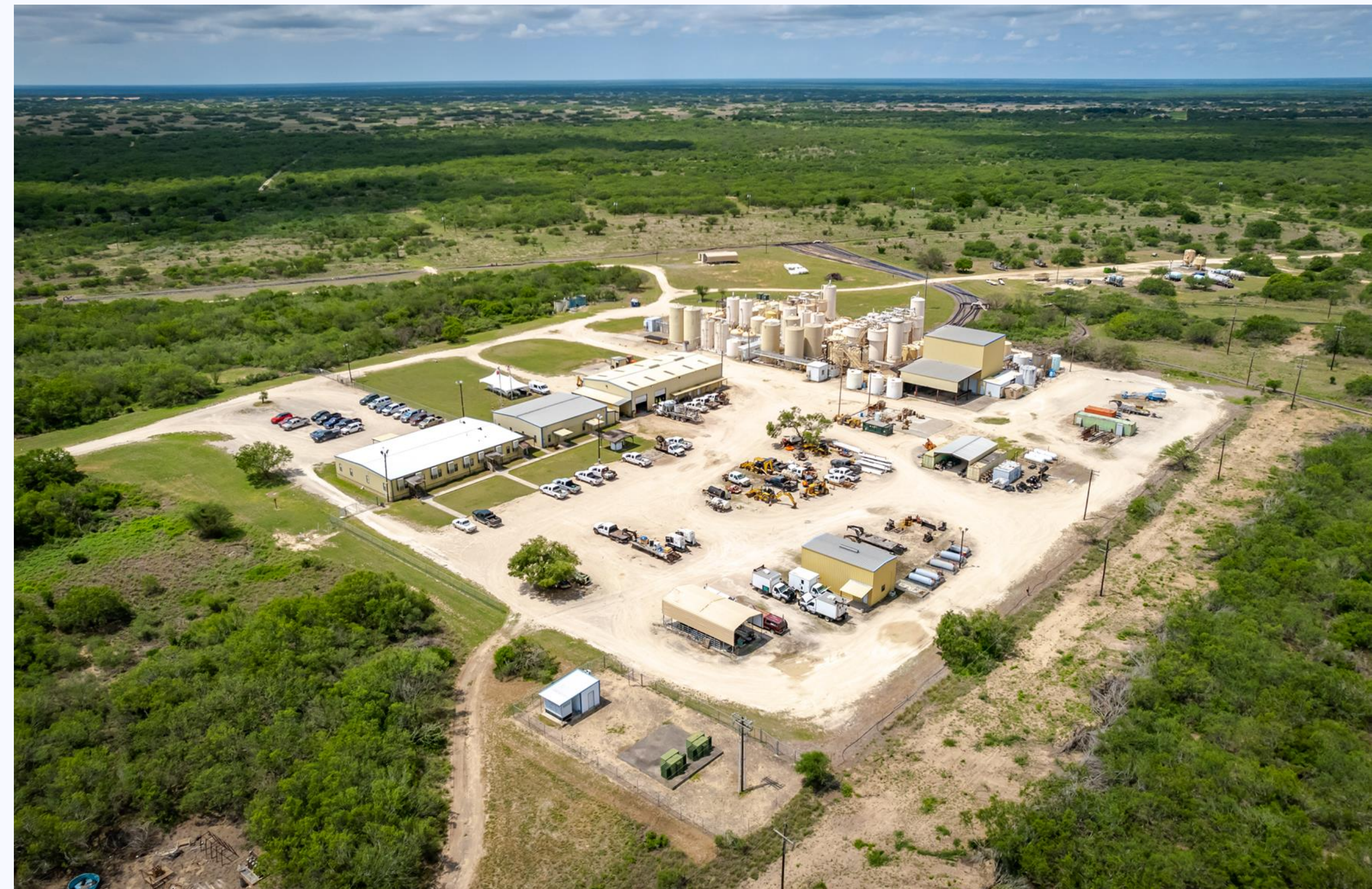
Alta Mesa Central Processing Plant
