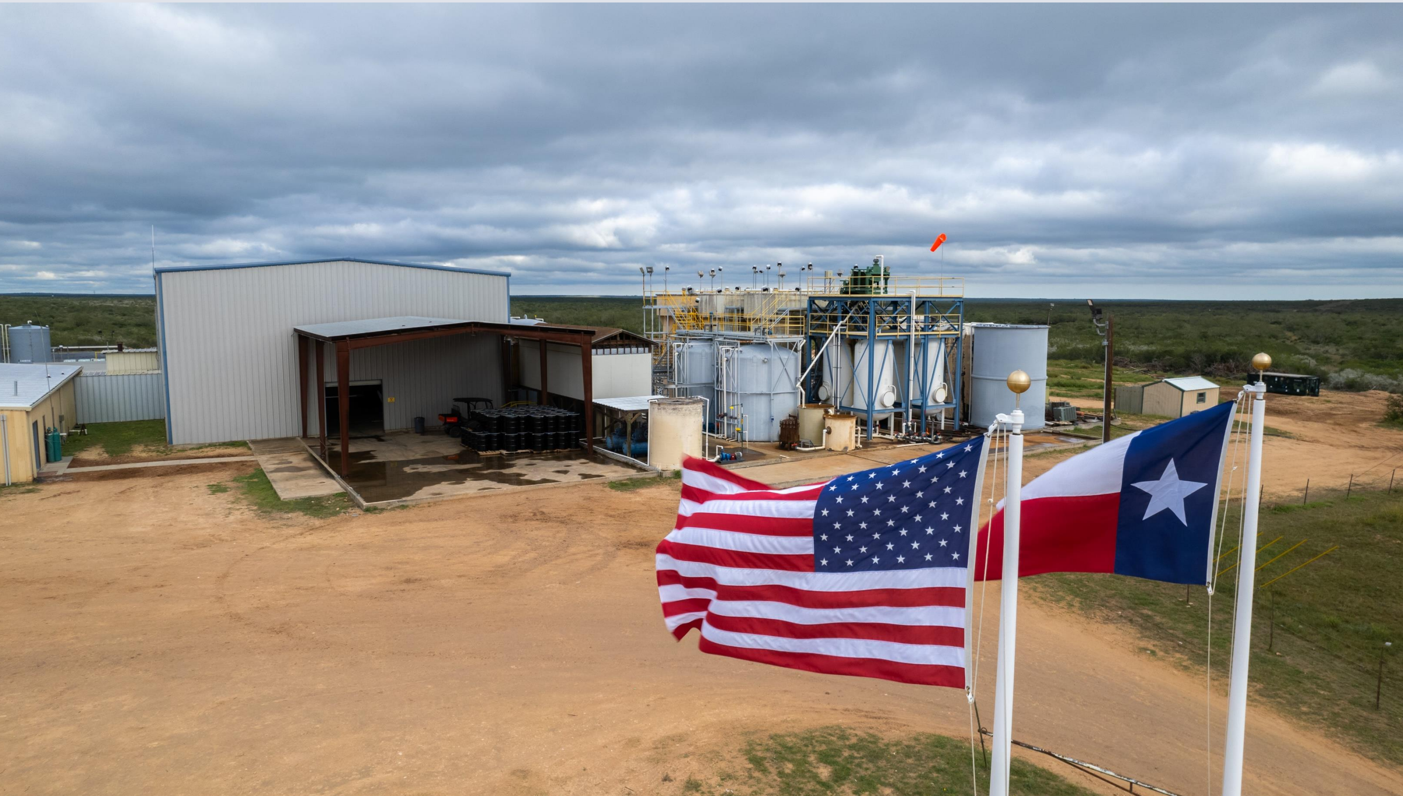
Rosita ISR Uranium Central Processing Plant
