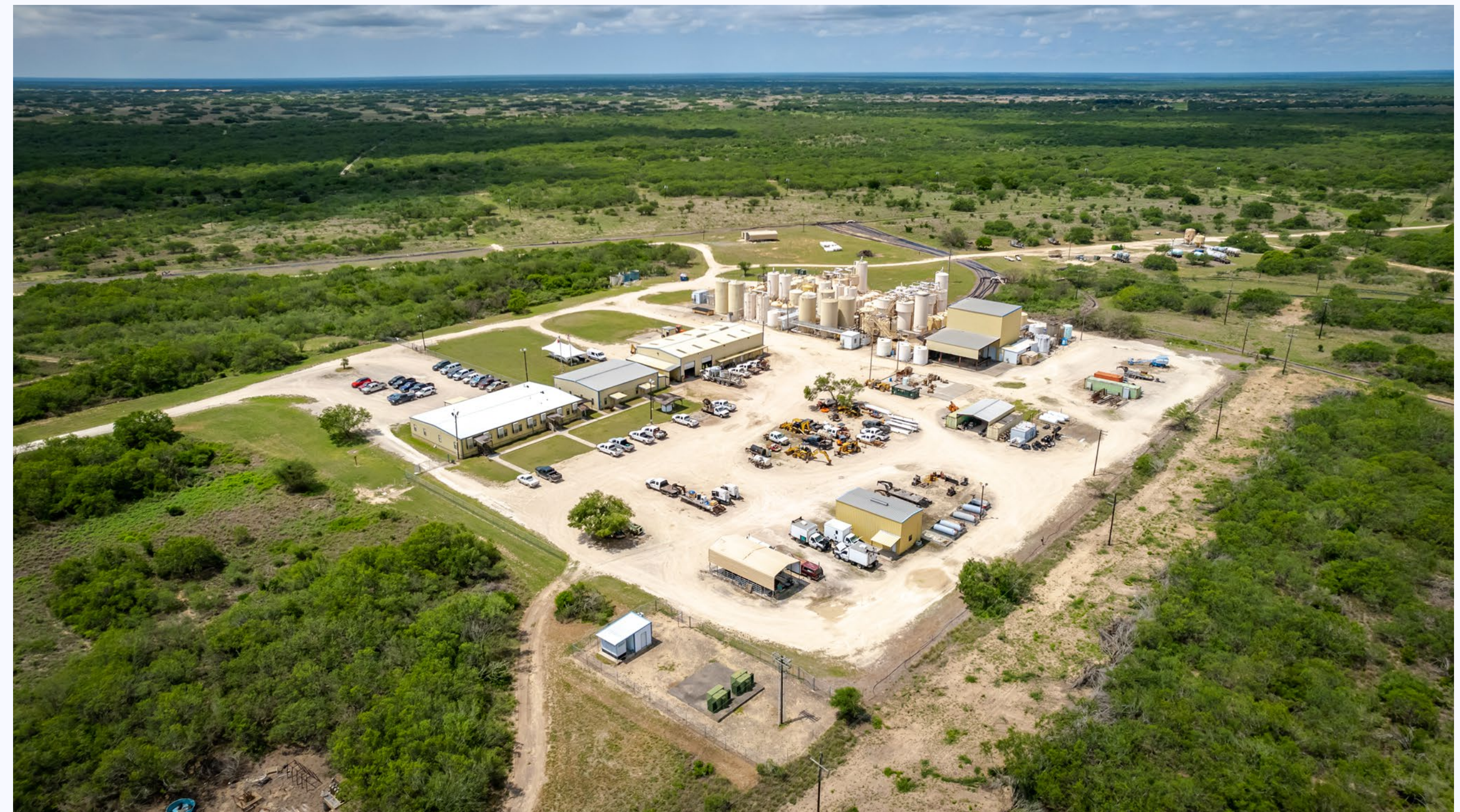
Alta Mesa Central Processing Plant
