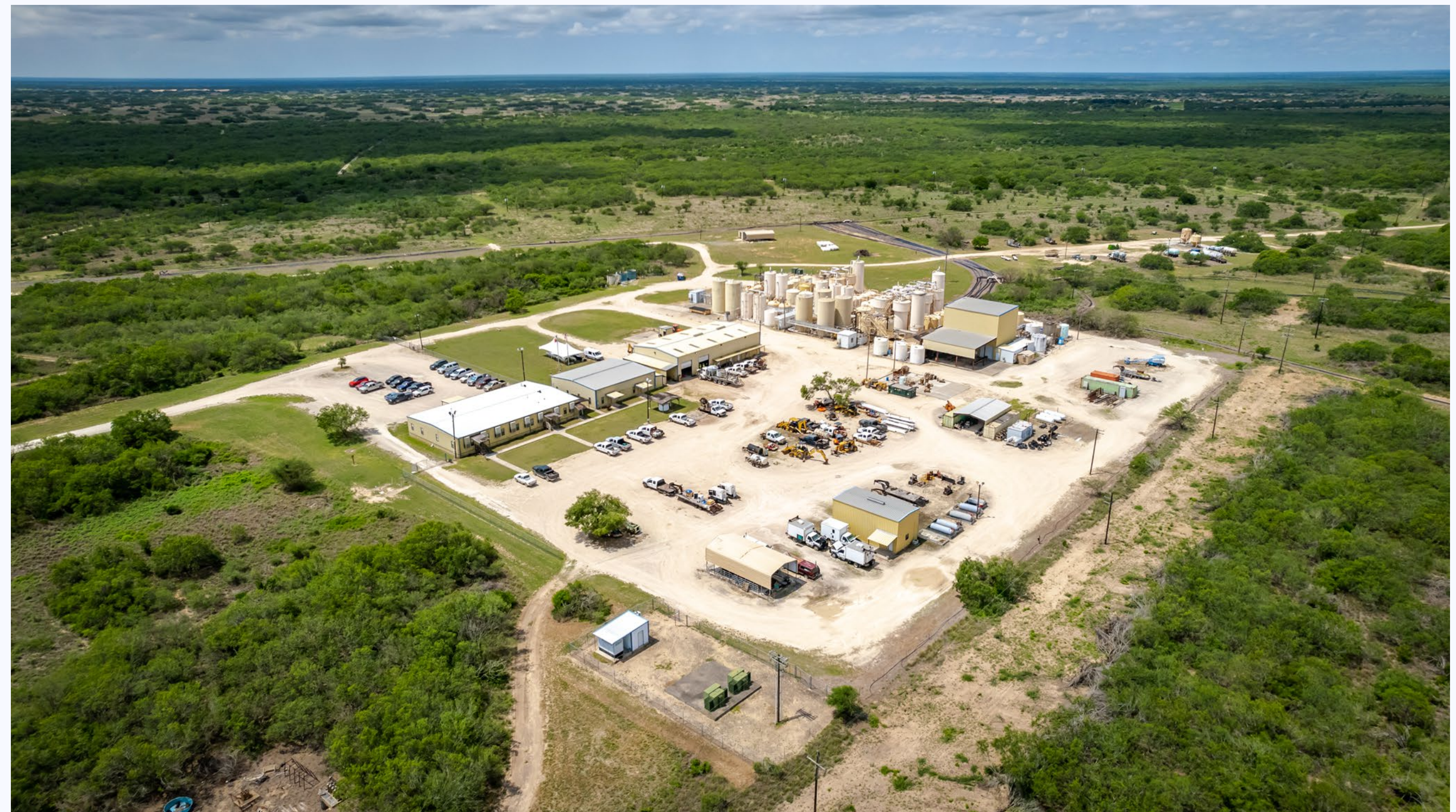
Alta Mesa Central Processing Plant
